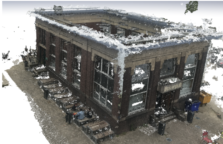
Figure 5.14: Example building captured by cellphone.
